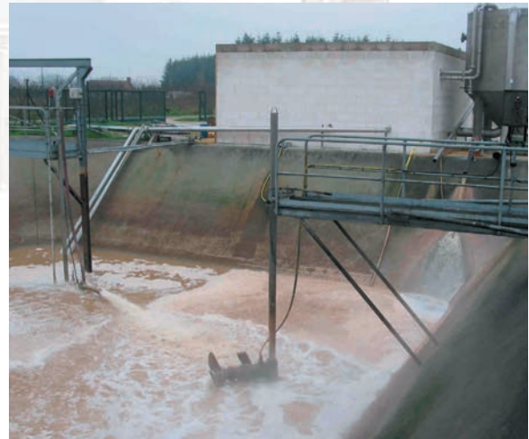
Combined system of submersible AirJet and submersible mixer in equalization tanks from vegetable processing industry
