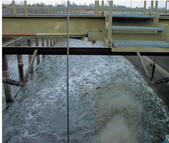
Storm water tank cleaning
