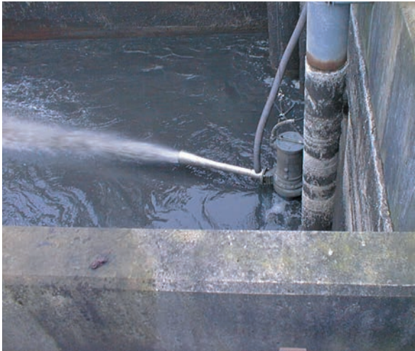
Storm water tank cleaning
