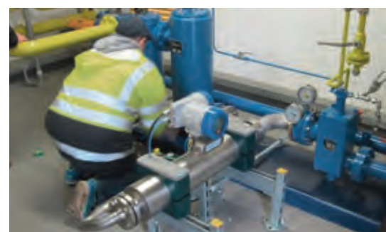
MID MI-005 tanker filling system for liquefied gas
