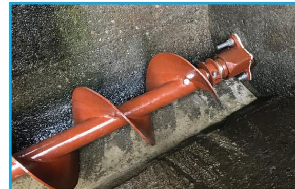
In lieu of standard chain and flight cross collectors, Brentwood can also provide our motorized chain driven screw conveyor assembly. Available in carbon steel and stainless steel in a variety of diameters, these augers consist of a rotating helical screw blade, or "flighting", that convey sludge collected from the longitudinal collector to a pit to be removed.
